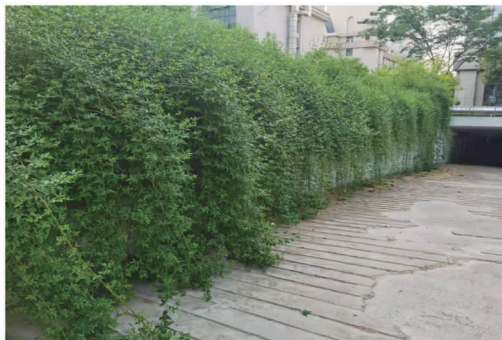
图 7 挡墙 Fig.7 Retaining wall
